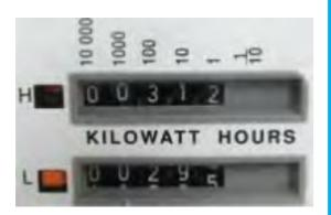
In this example, the meter shows two displays - H (High/Peak) and L (Low/Off Peak). Note some meters may have the H and L displays reversed. The reading for this example is H 0 - 0 - 3 - 1 - 2L 0 - 0 - 2 - 9 - 5
